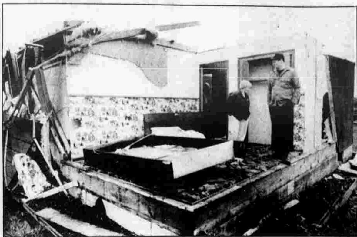
SURVEYING THE DAMAGE — Margie Sharo and her son, Kenny, stand in a bedroom of his Clarkson, Ky., home Thursday and survey the damage done by a tornado that hit the area Wednesday. Sharo, his wife, and two sons, fled to a crawl space under the house and waited for the storm to pass.
